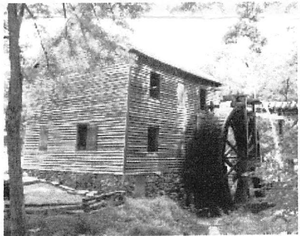
An old water powered grist mill typical of the type owned by Bartholomew
